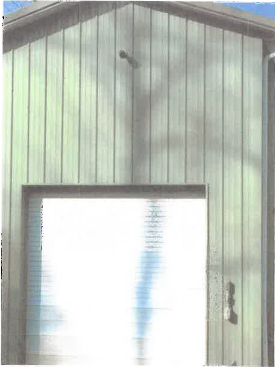
Figure 11 – Security camera on building over garage door.
