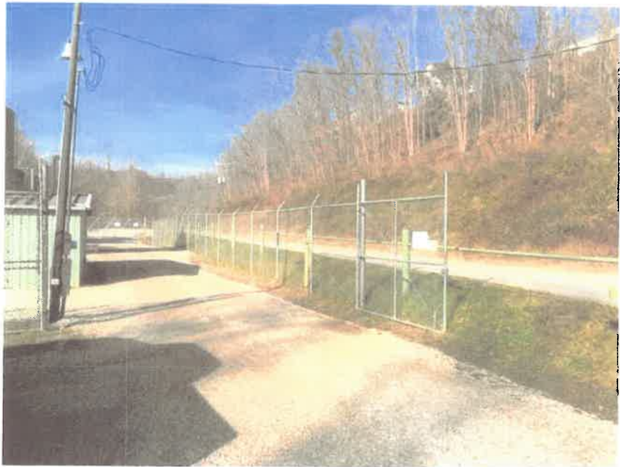
Figure 1 – Photograph of access road and gate to the Columbia Gas 20320 (Wallace Unit #1) injection well location and Tuppens Creek surface facility.
