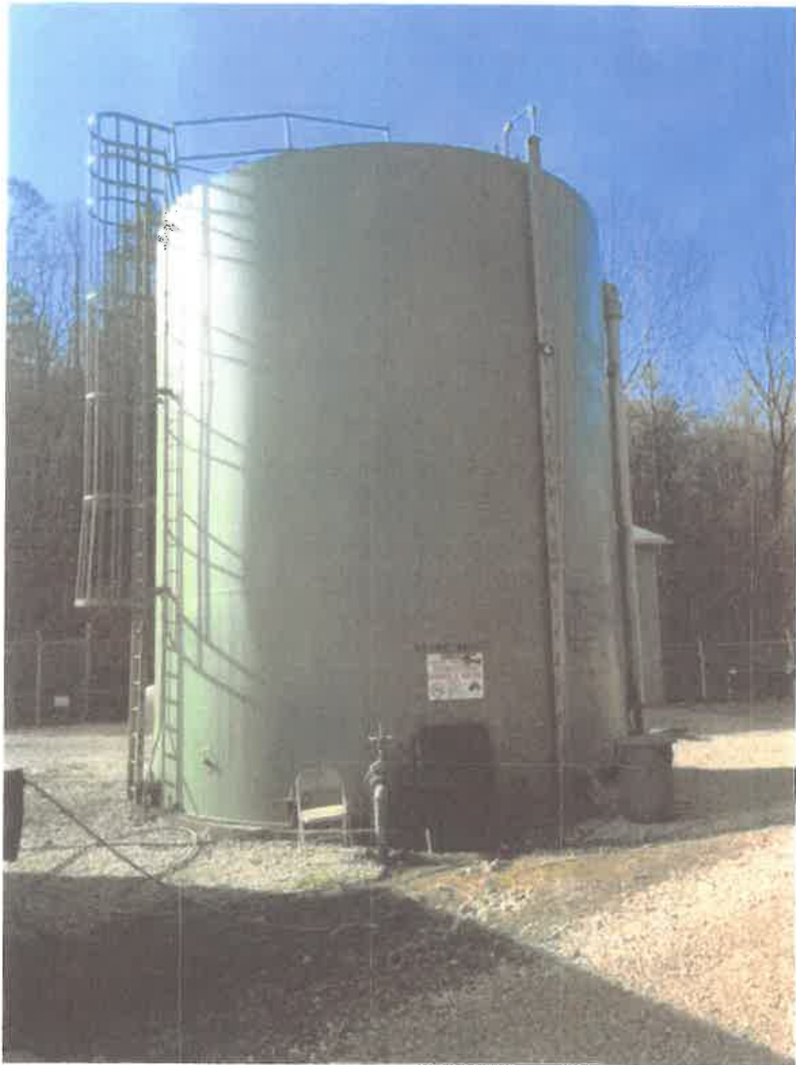
Received Office of Oil & Gas JAN 04 2016 Figure 6 – Double-walled large storage tank.
