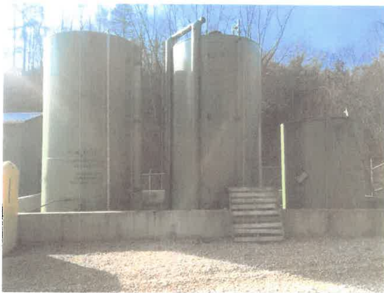
Figure 3 – Photograph of tank battery and concrete secondary containment at the Tuppens Creek surface facility.
